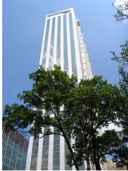
Figure 9: Modern day bank (Bank of America)
